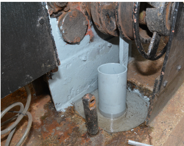
New anchor chain guide tubes
